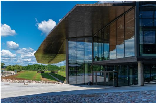
*Roof design challenge: Schöck Isokorb ensures thermal separation of the cantilevered roof, Photo: Laimonas Ciūnys*
