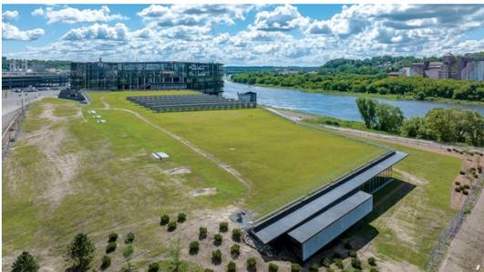
*The architects of E. Miliūno studija used the relief of the terrain for the design, which now flows smoothly into the single-story building in the form of a green roof.*
