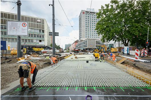
*The "lower layer" of the reinforcement immediately before completion.
