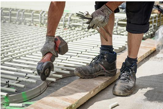
*The Combar reinforcing bars are cut to the correct length. Photo: Moritz Bernouilly*
