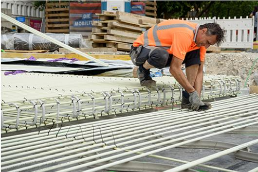
*Fixing the reinforcement with cable ties. Photo: Moritz Bernouilly*
