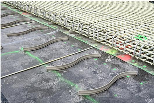
*Laying the spacers for compliance with the concrete cover. Photo: Moritz Bernouilly*
