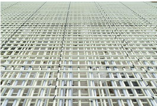
*View of a floor slab reinforced with Combar. Photo: Moritz Bernouilly*
