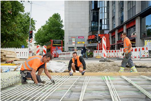
*Align the longitudinal bars according to the spacing prescribed in the reinforcement plan. Photo: Moritz Bernouilly*
