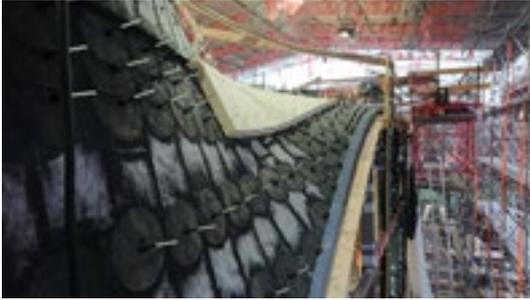
*The energy efficiency of the roof is ensured by 14 centimetres of thermal insulation and Schöck Isolink façade anchors, which minimise thermal bridges.
