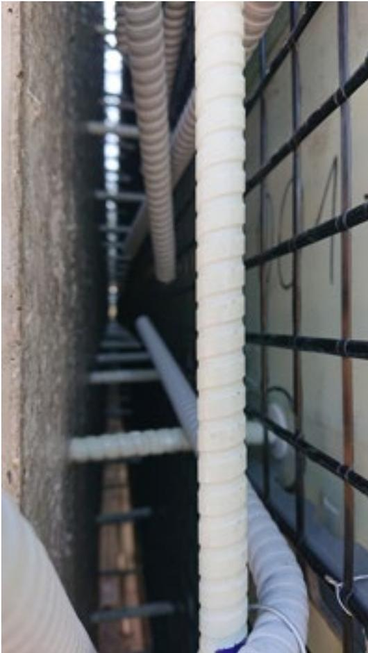
*To use Schöck Combar to reinforce walls at the corners, the required bending radii had to be adapted to the requirements of the slender wall structures.
