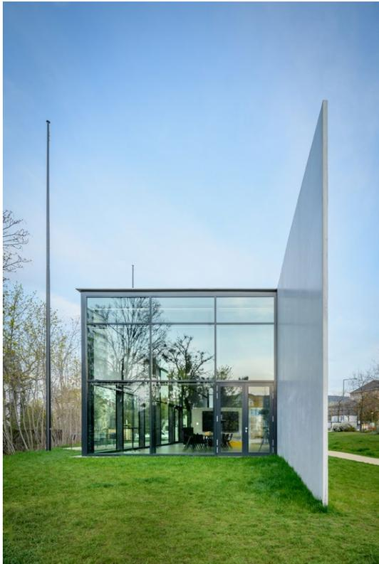
*The CUBE consists of two parts – the TWIST and the BOX. It is an experimental building and at the same time a vehicle for researching the long-term suitability of carbon concrete in terms of structural design, structural engineering and building physics.*
