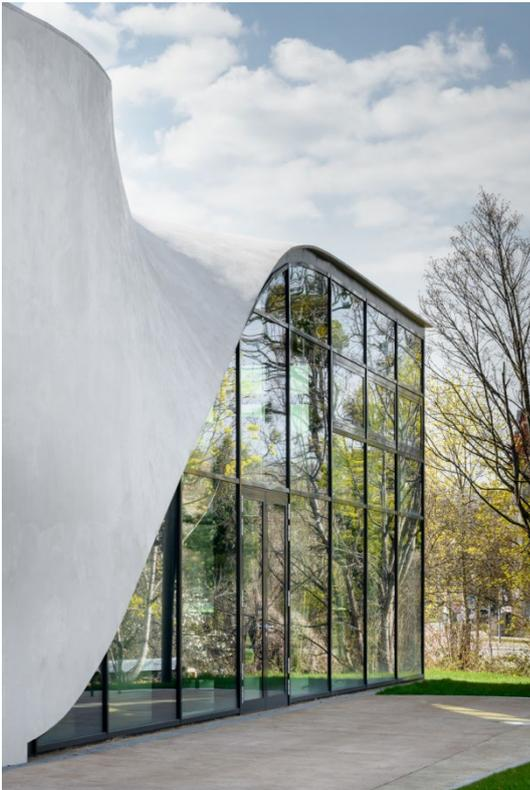
*The different shapes of the Combar® lent stability to the load-bearing structure unusual building geometry.*
