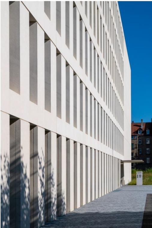
*Every façade component was sandblasted at the precast plant.
