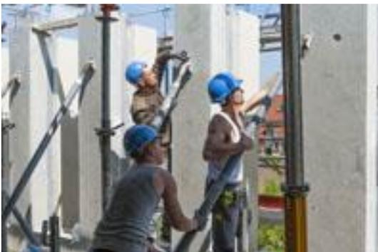
*The façade is made up of more than 350 precast concrete components, with variously designed individual elements with two to four shafts.*
